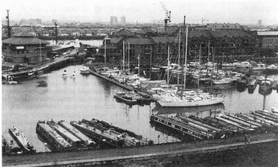
A view of the Limehouse Festival from the top of the Hydraulic Accumulator Tower, with the fleet of narrowboats moored to the "beach" and sailboards in action near the tidal lock.
